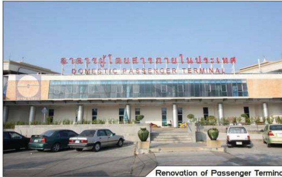
Renovation of Passenger Terminal
